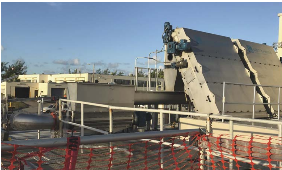
Figure 5. Owner-Furnished Screenings Equipment Under Installation
