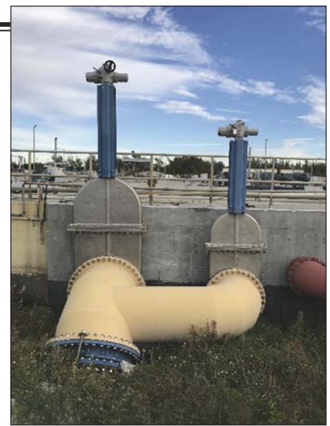
Figure 7. Special Prefabricated 48-in.-by-36-in. Connections at Plant 2
